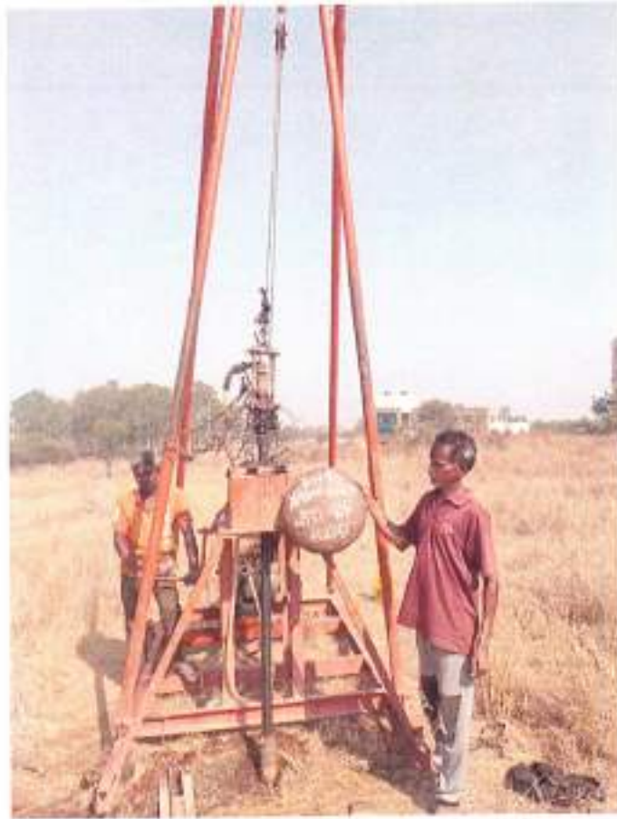
Borehole Drilling in Progress
