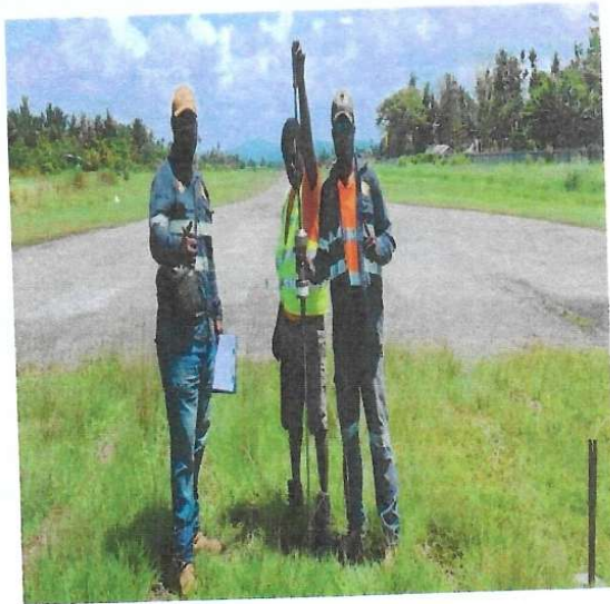
DOWH-MST BRANCH Geotechnical Engineer and team conducting DCP test at CH 00 – Start Point
