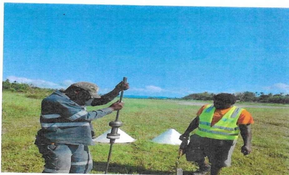
Figure 2. Geotechnical Engineer DOWH-MST Branch conducting DCP Tests at Chainage 00 – LHS of airstrip 10m from the edge of existing pavement (runway)
