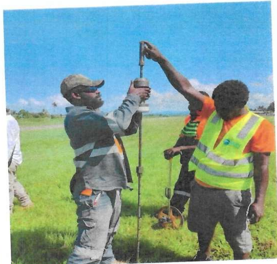
DCP tests conducted at CH400 by MST Geotechnical Team and NAC representative.
